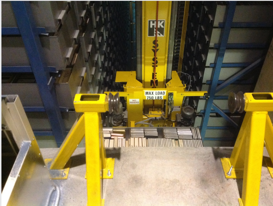
An automated robot library system at San Francisco State University.
